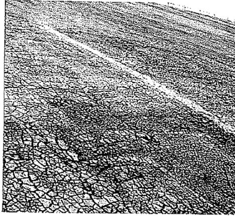
**Figure 2: Hairline cracking on bituminous concrete facing dam leading to score 6 given to the watertightness component protection function**
