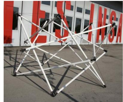
Figure 12 Folding tensegrity ring. 2007. Motro et al.
