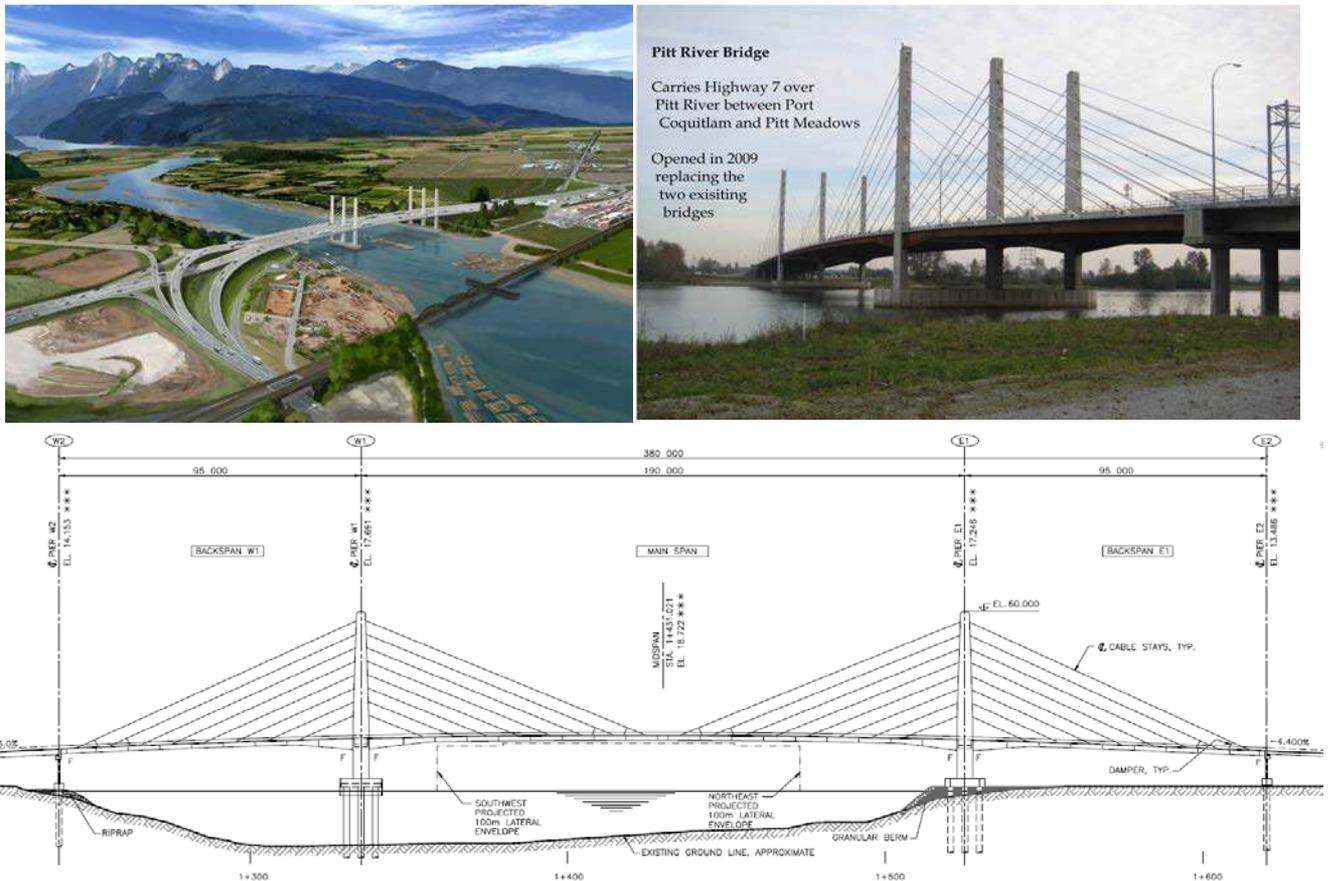
Figure 1. Overview and Schematic elevation of Pitt River Bridge<sup>4</sup>
