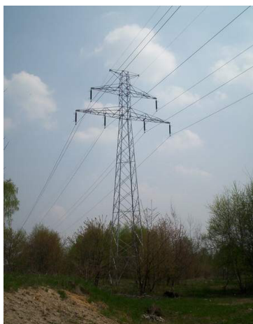
Figure 1 : Suspension tower type M52.
