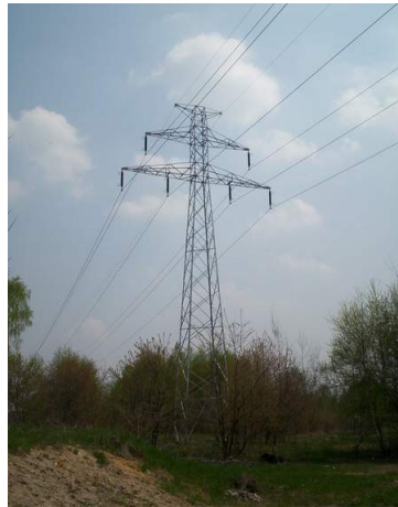
Figure 1 : Suspension tower type M52.
