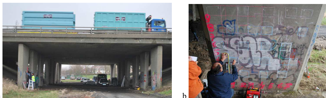
Figure 5: Marly's bridge: a – Global view – b – Zoom on S-pile
