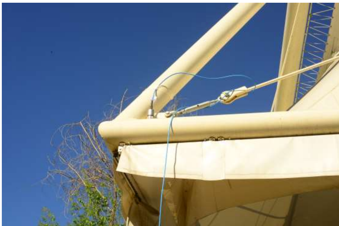
Figure 5: Sensors in field vibration test
