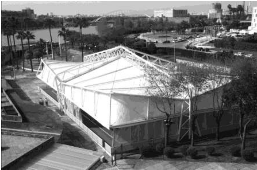
Figure 2: Aerial view of the roof with partially open side
