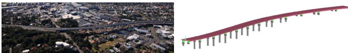
Figure 2: Newmarket Viaduct (left) and its 3D FE model (right).
