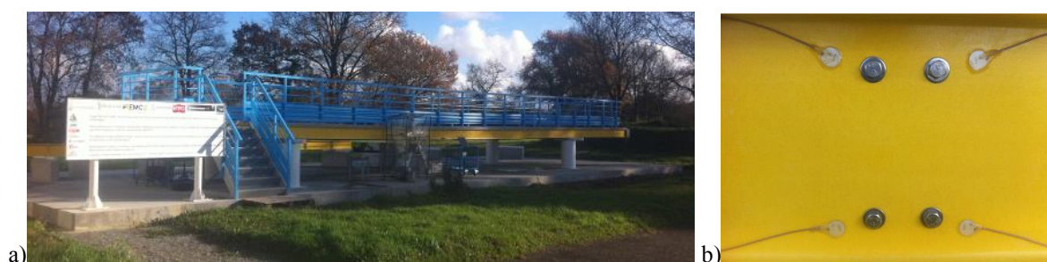
Figure 10: a) Demonstrator composite Footbridge; b) Miniatures sensors for bolt assembly monitoring.
