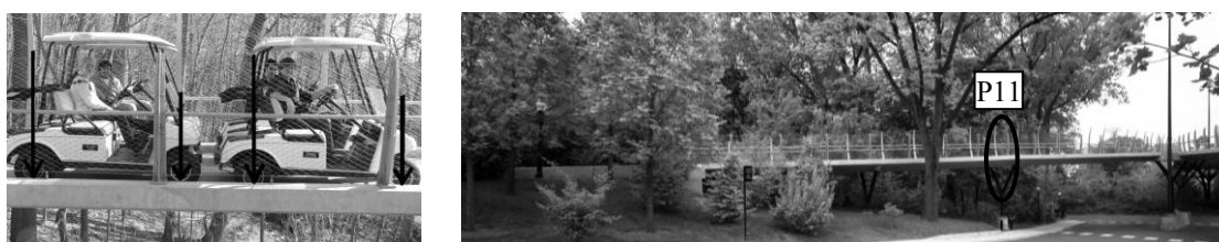
Figure 2: Left: Load test, the bridge was loaded with four golf carts. Right: Location P11 is above a support.
