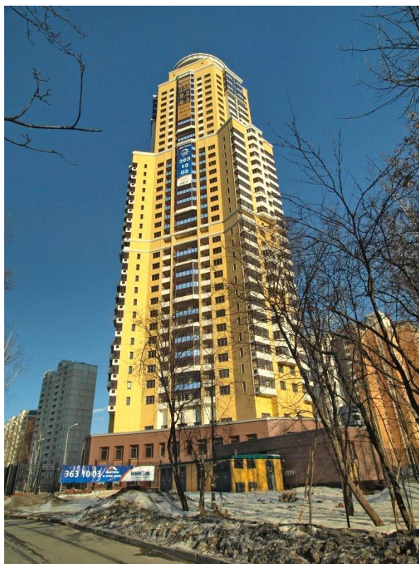
Figure 1: 43-storey apartment at Dybenko, 38 in Moscow
