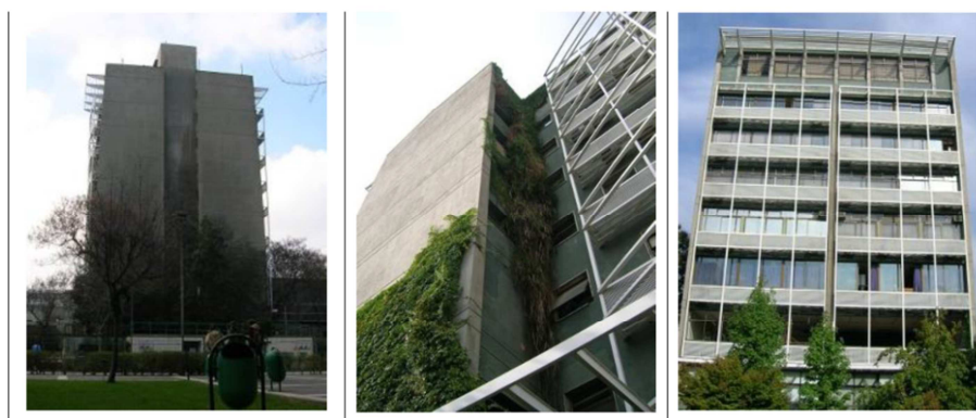
Figure 1: Central Tower - General Views.
