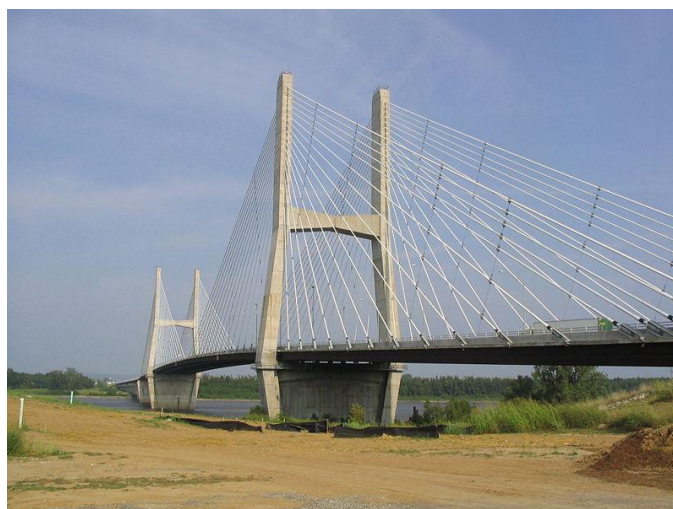
Figure 2: The Bill Emerson Memorial Bridge (Framerotblues, 2007; with permission)
