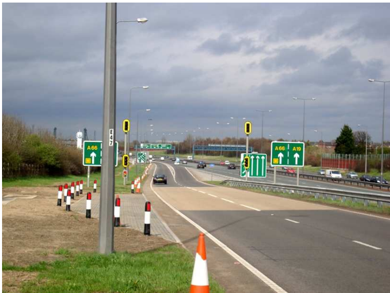
Ramp metering on the A19 in Middlesbrough, UK.
