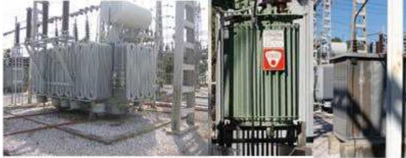
**Fig. 2.** Protected substation components: HV/MV Power Transformer (left), Neutral Reactance (centre) and Neutral Resistor (right).
