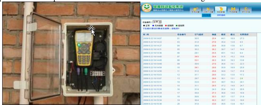
Fig. 6. Test and real time data pictures
