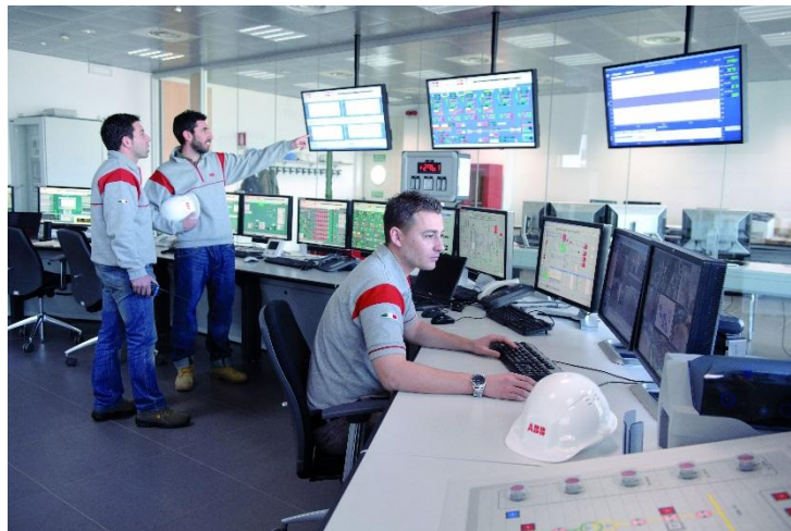
Fig. 1. Illustrative photo of a control room with operators and their workstations running applications with HMI (Source: A photo from a project)
