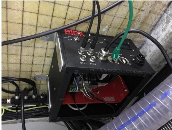
**Fig. 2.** The Universal Marine Gateway as implemented on final Hydrolift P-42 prototype
