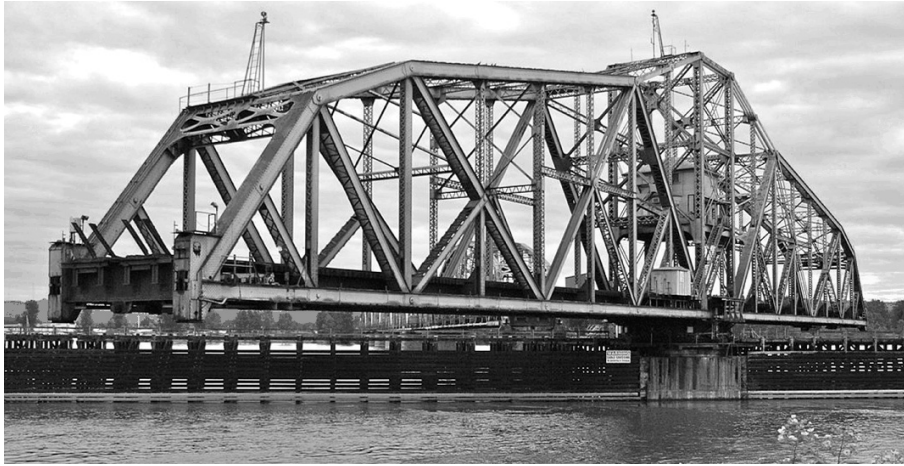
Figure 1. An open BNSF railroad swing bridge [18].
