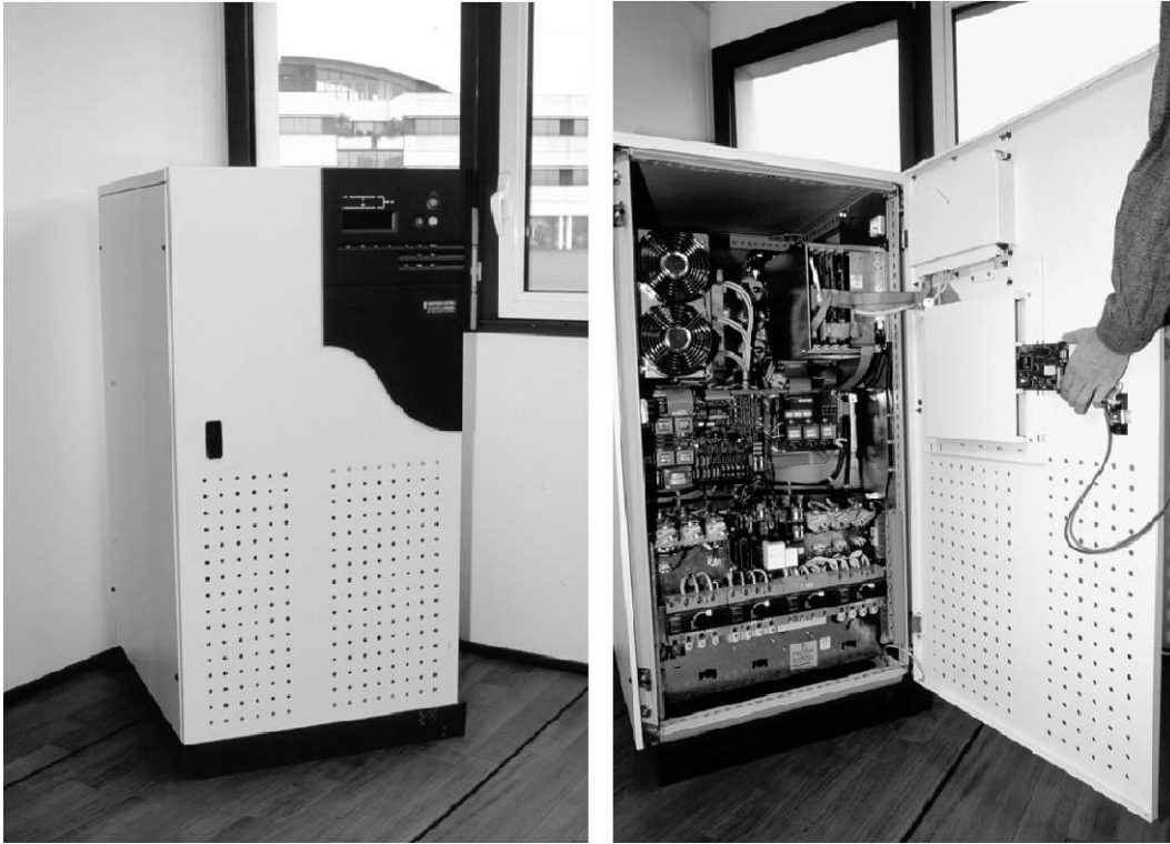
Figure 2: Outside and inside view of an UPS (picture courtesy of MGE-UPS).
