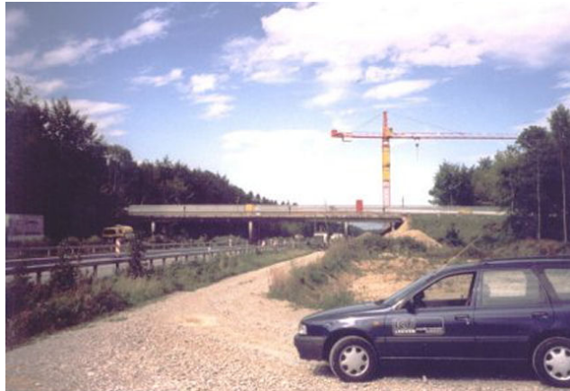
Figure 2: Photo of the Z24 bridge.
