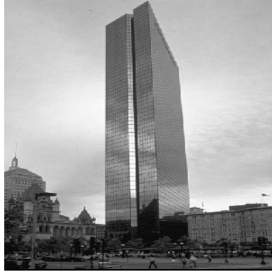
(a) John Hancock Tower, Boston.
