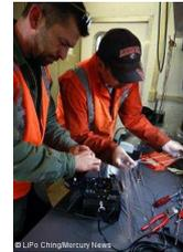
**Fig. 1.** Crew splicing fiber-optic cables.
