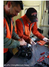
Fig. 1. Crew splicing fiber-optic cables.
